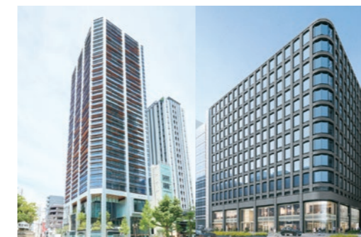
Midosuji Daibiru Building Construction completed in January 2024 Yaesu Daibiru Building Construction to be completed in mid 2025
