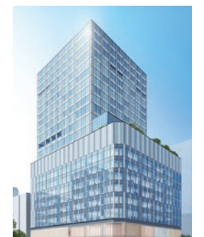
Sapporo Daibiru Building Construction to be completed in January 2027
