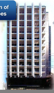
Estate Yodoyabashi (SANCOINN OSAKA YODOYABASHI)
