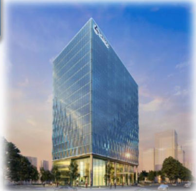
Starlake Area Redevelopment Project (Hanoi, Vietnam)
