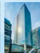
The Akihabara Daibiru Building
