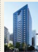
The Hibiya Daibiru Building
