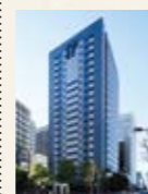
The Hibiya Daibiru Building
