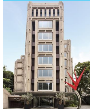
Kojimachi Daibiru Building
