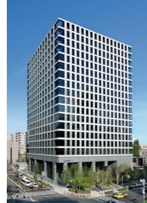
Tosabori Daibiru Building
