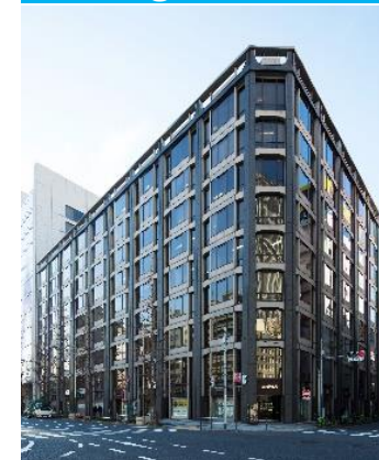
Yaesu Daibiru Building
