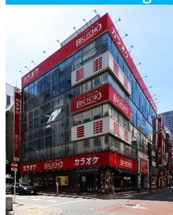
Nihonbashi 3-Chome Building
