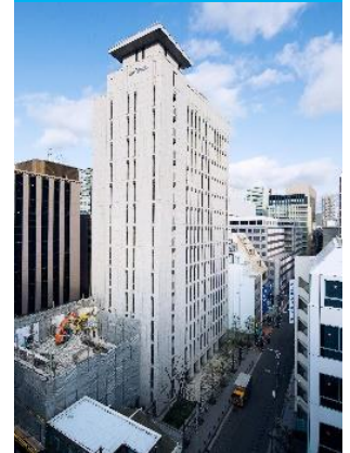
Yodoyabashi Daibiru Building
