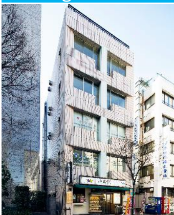
Estate Shiba Building
