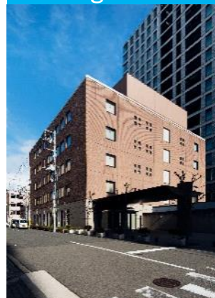
Estate Tosabori Building
