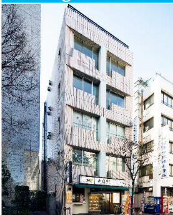
Estate Shiba Building
