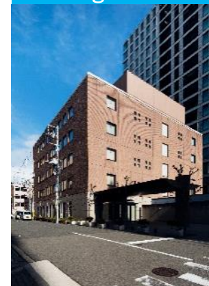
Estate Tosabori Building
