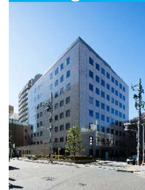
Shiba Daibiru Building
