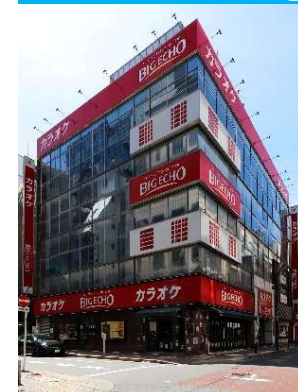
Nihonbashi 3-Chome Building
