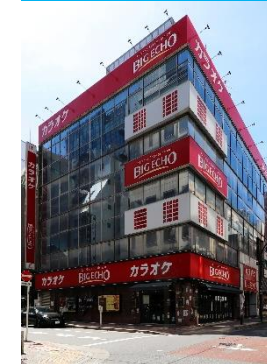
Nihonbashi 3-Chome Building
