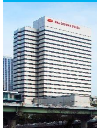
Dojima Daibiru Building (ANA Crowne Plaza Osaka)
