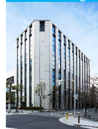
Kita-Umeda Daibiru Building
