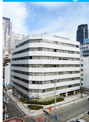
Awajimachi Daibiru Building
