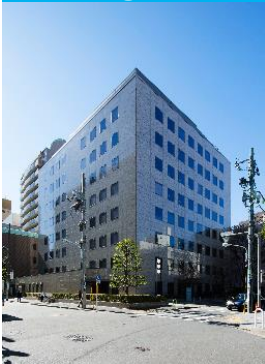
Shiba Daibiru Building
