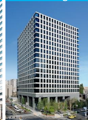
Tosabori Daibiru building
