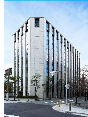
Kita-Umeda Daibiru Building
