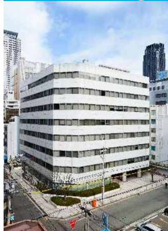
Awajimachi Daibiru Building
