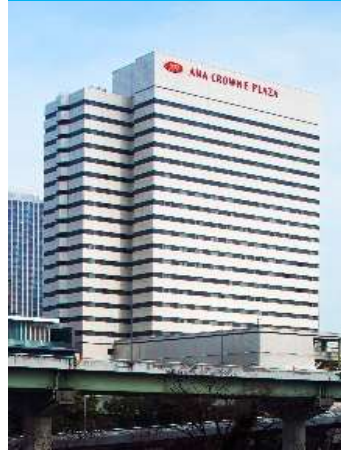
Dojima Daibiru Building (ANA Crowne Plaza Osaka)
