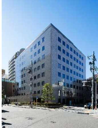
Shiba Daibiru Building
