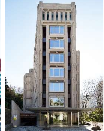
Kojimachi Daibiru Building
