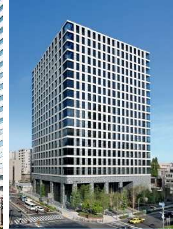
Tosabori Daibiru building
