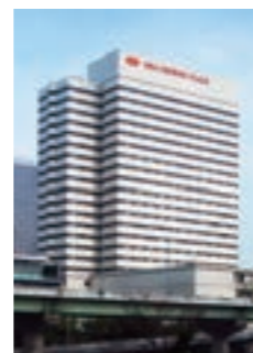
Picture 5 Dojima Daibiru Building
