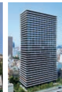
Picture 14 Shin-Daibiru Building
