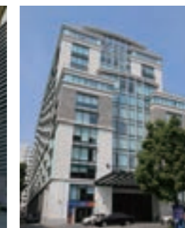
Picture 13 CornerStone Building
