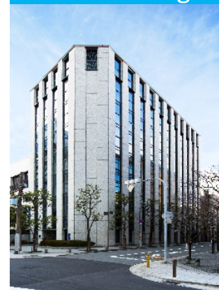
Kita-Umeda Daibiru Building
