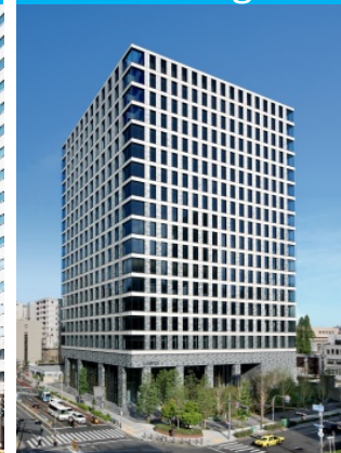
Tosabori Daibiru building
