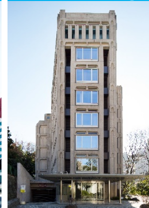
Kojimachi Daibiru Building
