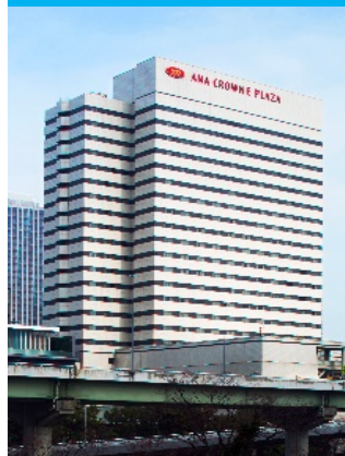
Dojima Daibiru Building (ANA Crowne Plaza Osaka)
