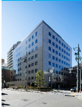
Shiba Daibiru Building
