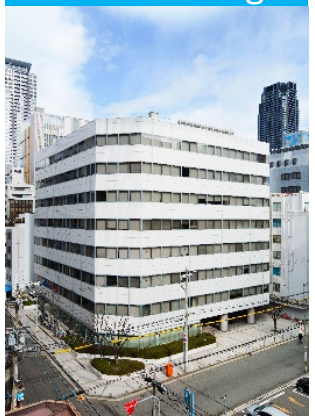
Awajimachi Daibiru Building
