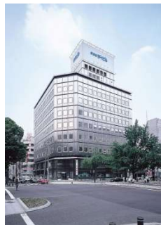
Midosuji Daibiru Building
