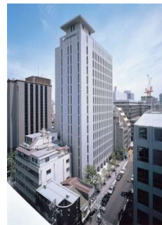
Yodoyabashi Daibiru Building
