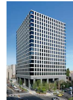
Tosabori Daibiru building
