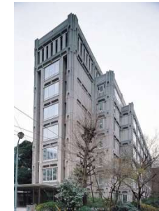
Kojimachi Daibiru Building
