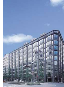
Yaesu Daibiru Building
