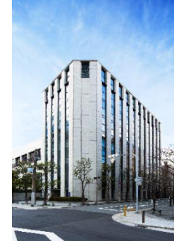
Kita-Umeda Daibiru Building
