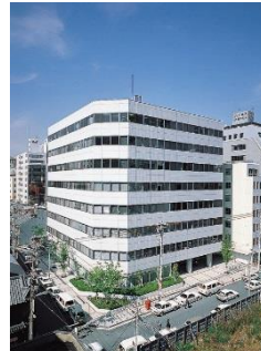
Awajimachi Daibiru Building
