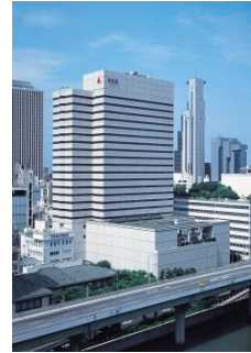
Dojima Daibiru Building (ANA Crowne Plaza Osaka)
