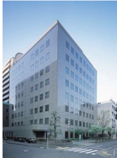
Shiba Daibiru Building
