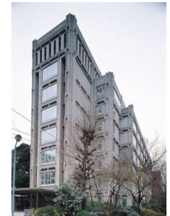
Kojimachi Daibiru Building
