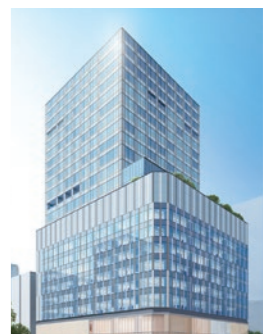
Sapporo Daibiru Building Construction to be completed in January 2027
